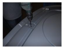
b) Into these holes will be inserted two cylinder head screws M8 x 35 mm (19771) and the two large washers (20058).
